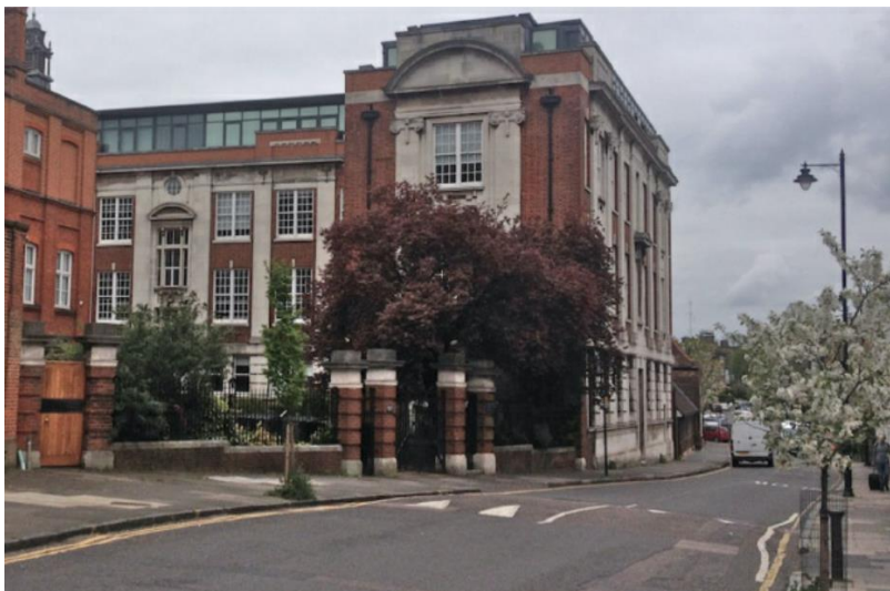
Figure 9: Existing Science Block
